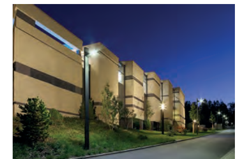
Kurhaus, Bad Alexandersbad
